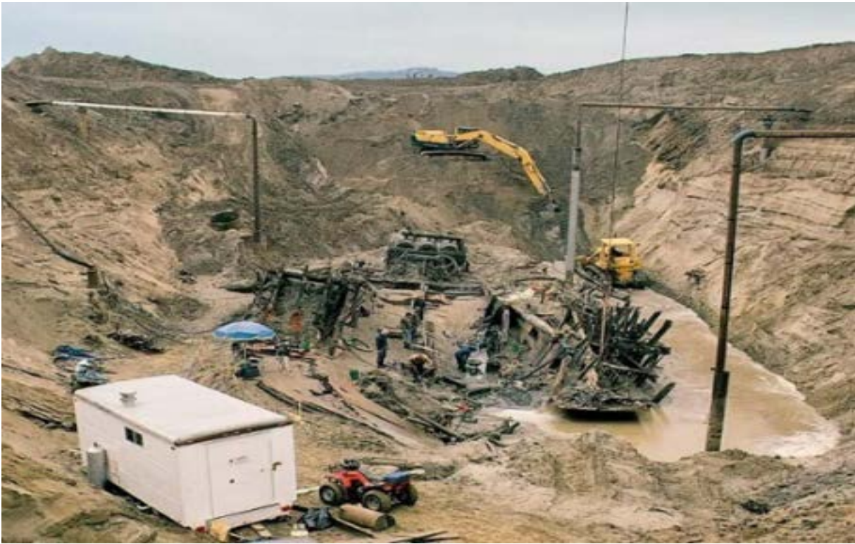
The excavation site
